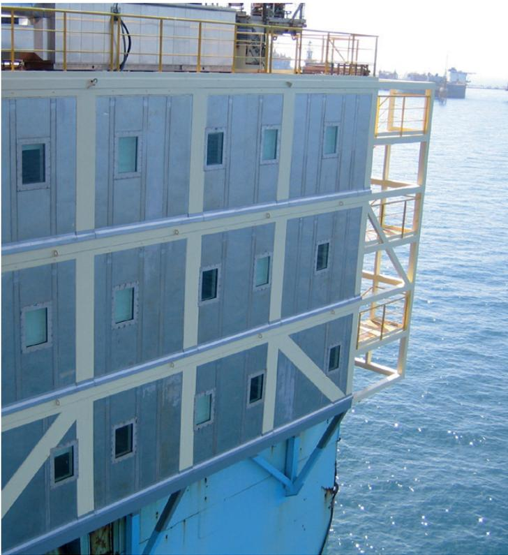
External Blast Wall Cladding
